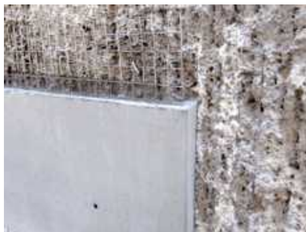
Fig. 8. Layer of concrete.
